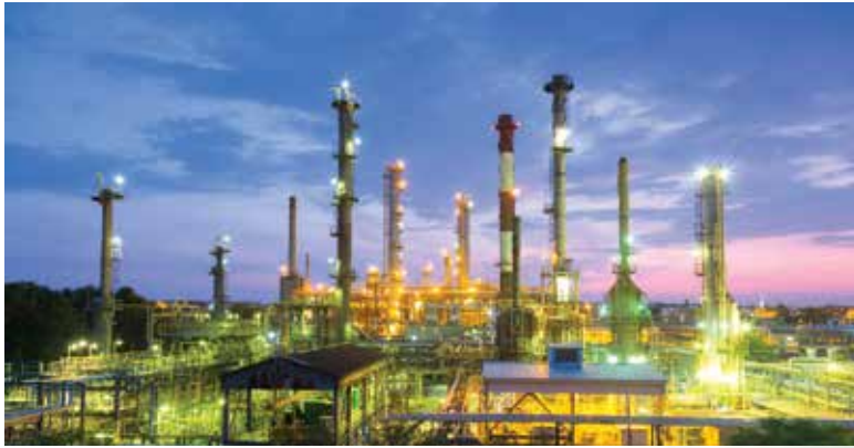
Attock Refinery Limited, Morgah, Rawalpindi
