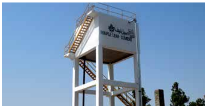
Development of Daud Khel Water Supply Scheme
