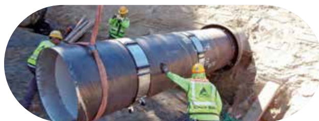
Steel line pipes are primarily used in transmission pipelines in the oil, gas, and water sectors. These line pipes are also used in construction, usually as piles at ports and jetties.
